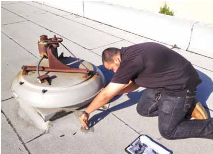
› A CIS Technician measures an equipment curb during a roof inspection. Photo courtesy of CIS.
